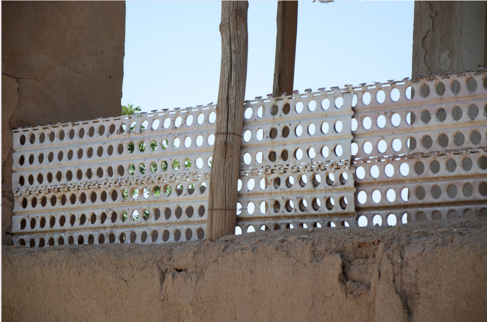
Picture by: Shahram Khosravi Pierced steel planks as balcony railing Bakhtari, Southwestern Iran
